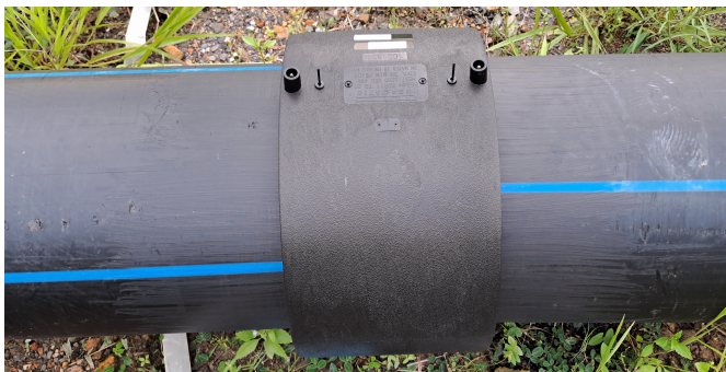
Figure 12: A HDPE pipe joint
