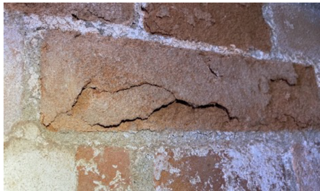
Figure 2: Bricks with peeling due to salt weathering
