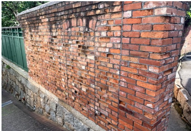
Figure 1: Buildings showing signs of deterioration due to salt weathering
